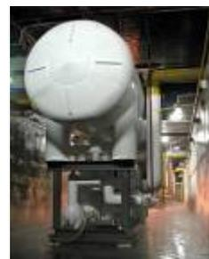
2. Stainless Steel Evaporative Condensers were used to withstand the tough ambient air and very high Hardness Water quality. However, water treatment and bleed off control are still essential to maintain the cooling water in good condition as much as possible.
